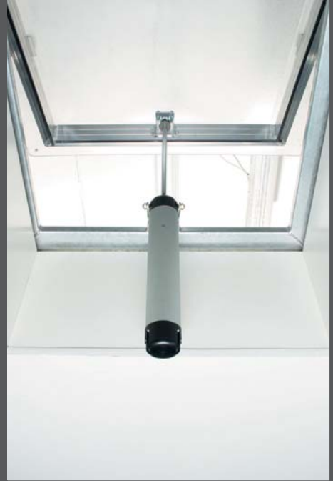
Installation on dome with fixing end brackets included
